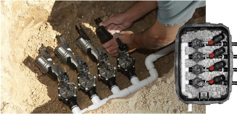
Rain Bird Control Zone Kits provide all of the components necessary for on/off control, filtration, and pressure regulation in one single package—making them simple to order and easy to install.
