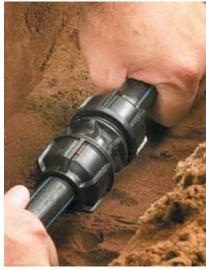
**3. Pipe Insertion**Insert the pipe until the stop is felt.
